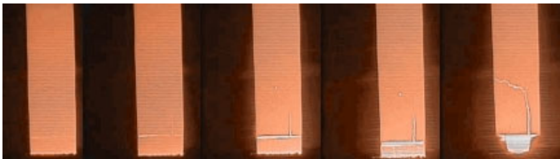
Figure 3. A lower column connection – loosening, crack propagation, and eventual stub-end loss over time.
