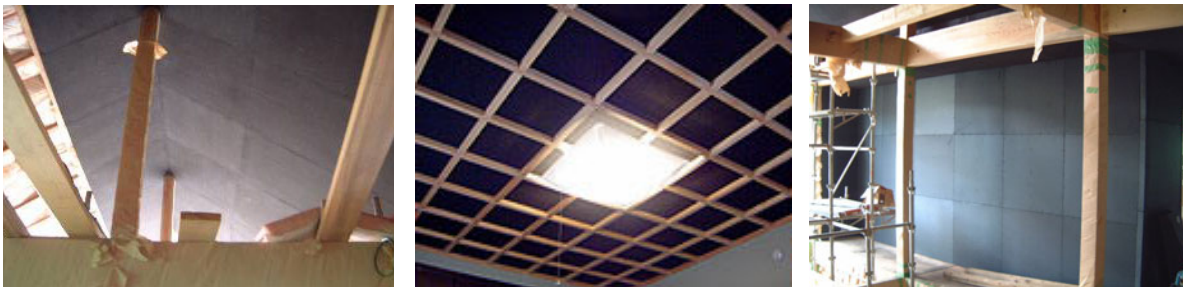
Figure 1. Construction examples. The charcoal boards masked with Japanese paper was used for wall.
