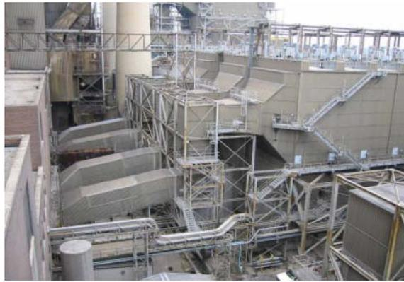
Figure 2. Portion of Ductwork and ESP of St. Clair Plant
